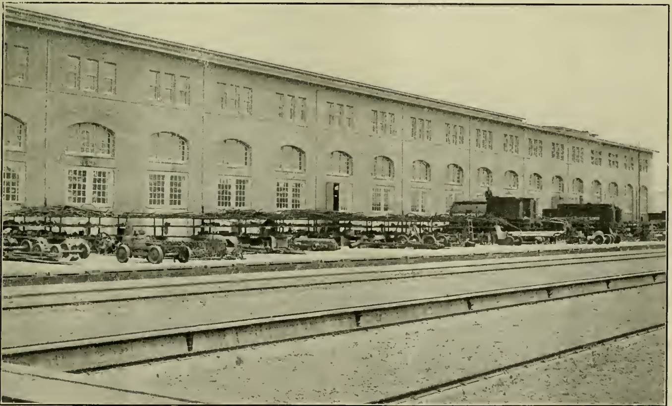
Bay Shore Shops of Southern Pacific Company Showing Racks for Storing Parts Removed from Locomotives Undergoing Repairs
